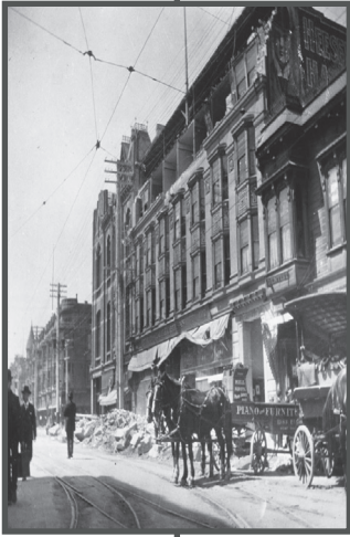
Photo: Earthquake damage, Washington Street, west side, April 1906.
