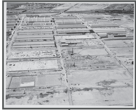
WWII Wartime Boom Photo: Aerial view of the Oakland Naval Supply Center under construction, June 11, 1942.
