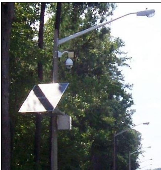
Through ongoing efforts to “go green” the City has installed solar powered street lights to increase energy efficiency.
