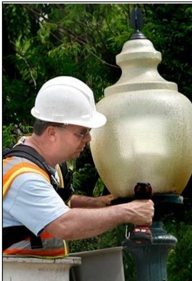
An Engineering employee installs LED street lights in Hilton Village of Newport News through one of the City’s first projects implemented under the EECBG grant. The projected savings from this retrofit is a reduction in energy cost by 60%. Image Source: Daily Press
