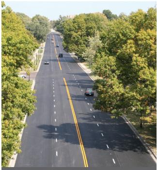
Santa Fe Boulevard in Overland Park, KS, was marked with wide outside lanes following resurfacing. Bicycle lanes will be marked when a subsequent project provides a link to another bikeway.
