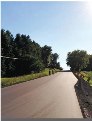
A paved shoulder has been added to Whalen Road in Fitchburg, WI, in uphill directions as part of a resurfacing project; markings have not yet been added.
