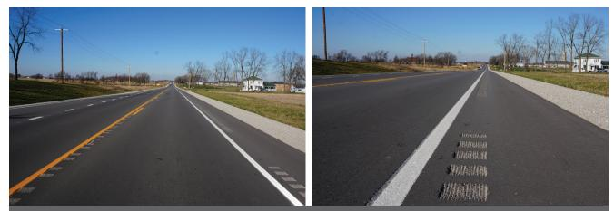
Highway 26 near Rosendale, WI, was recently resurfaced with 5-foot wide shoulders and narrow rumble strips that leave four feet of clear pavement to the right of the rumble strip.
