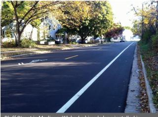
Bluff Street in Madison, WI, had a bicycle lane installed in the uphill direction and shared lane markings in the downhill direction during a resurfacing project. This configuration allowed parking to be preserved on one side of the street.
